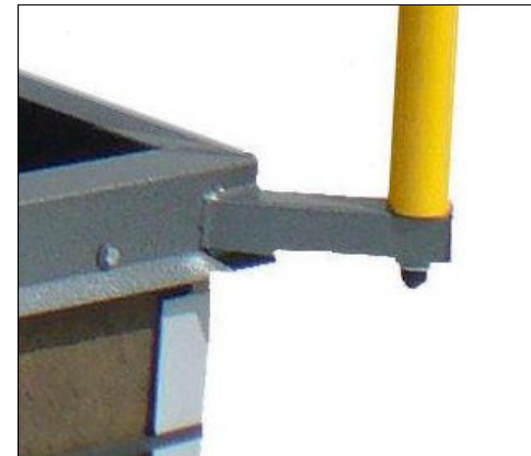
Rail Supports are Welded to Curb
