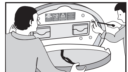
D. Install unit using screws and washer supplied
